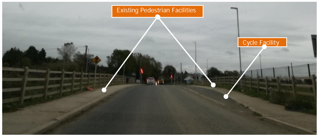
Figure 2.5: Existing Pedestrian & Cycle Facilities on the R125 Road Corridor
